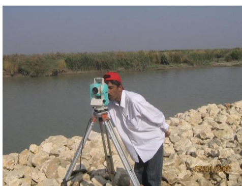
Total station work on the Barrage Bank
