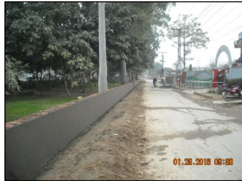
Plaster on boundary wall
