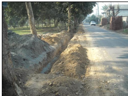
Excavation for boundary wall
