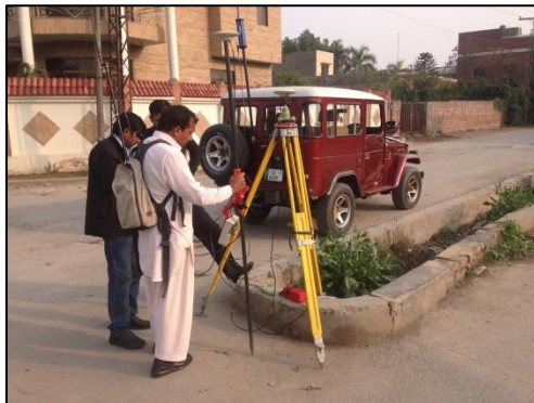
Checking of existing survey
