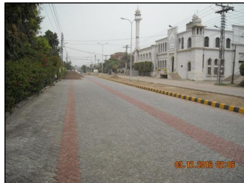
Brick paver and curbstone on road
