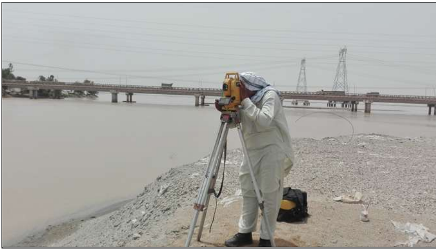
Topo survey work in progress at Indus River crossing
