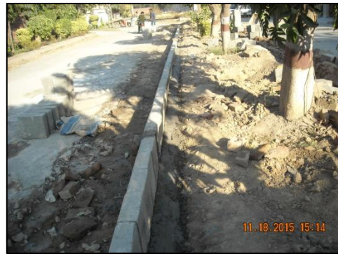
Installation of curbstone
