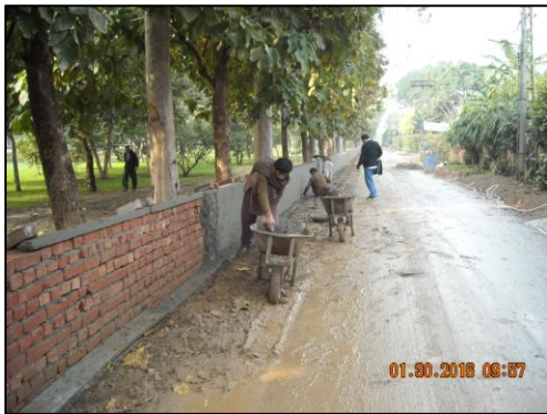
Plastering on wall in progress
