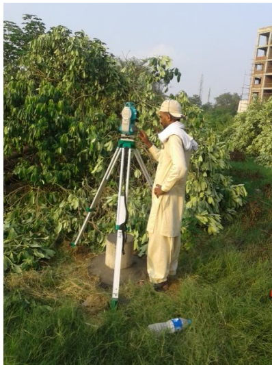
Surveyor at BM3 with Total Station
