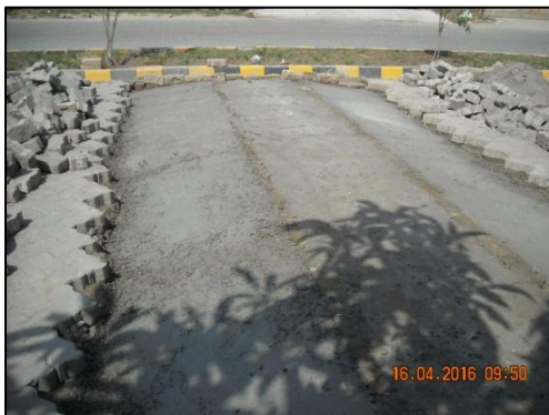
Construction of speed breakers
