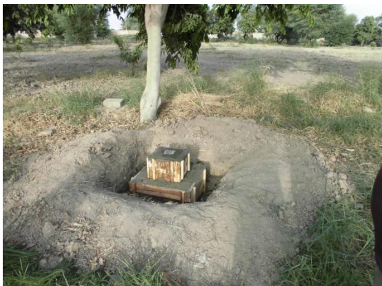
Permanent BM Construction WOTS-2
