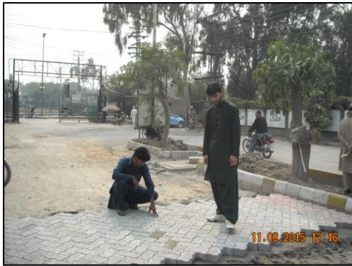
Brick paver installation in progress
