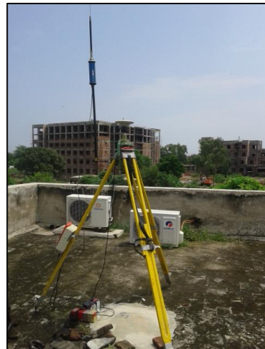
GPS base setup at site at CP2
