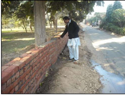
Wall Construction in progress
