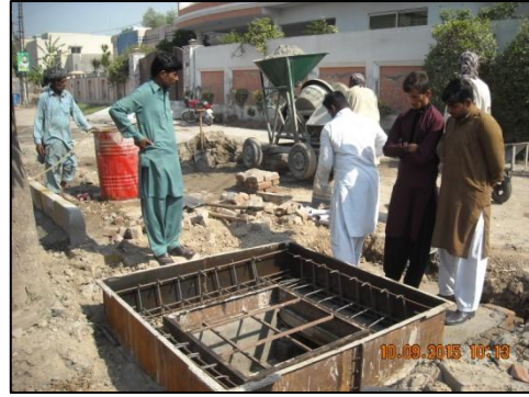
Formwork for large drainage inlet
