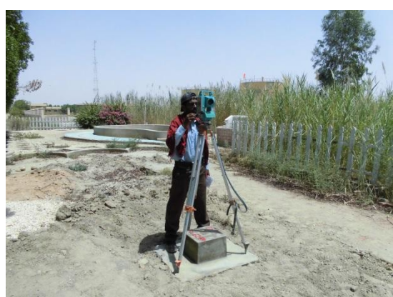
Survey Work in progress at WOTS-2
