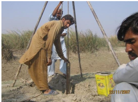
Manual boring for soil samples
