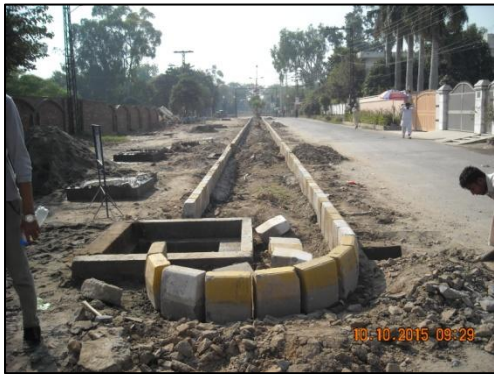
Installation of curbstone around median
