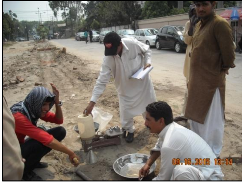
Soil compaction test in progress
