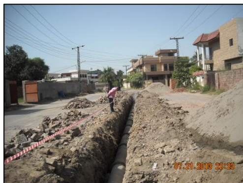
Excavation for concrete pipe
