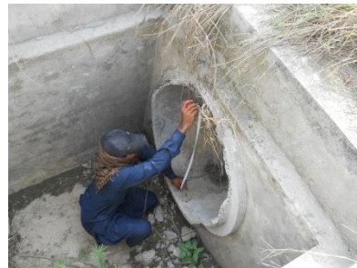
Pipe Measurement in Manhole
