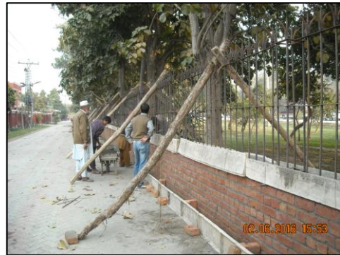
Installation of metal fence on wall
