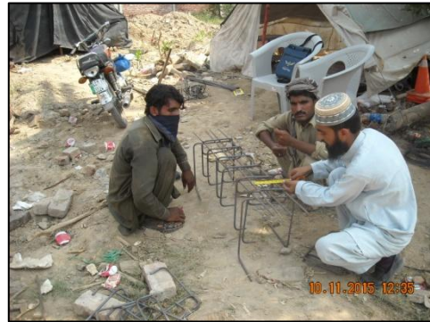
Verification of steel reinforcement
