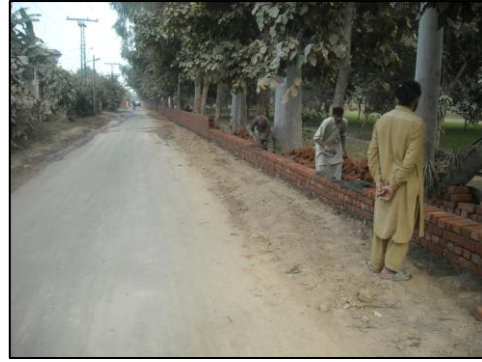
Wall Construction in progress
