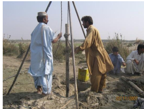
Manual boring for soil samples
