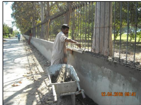
Installation of metal fence on wall
