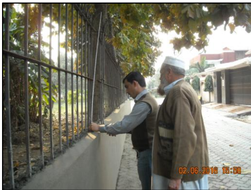
Checking of metal fence on wall
