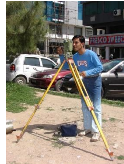
Instrument being set up for measurement of NIC Bldg
