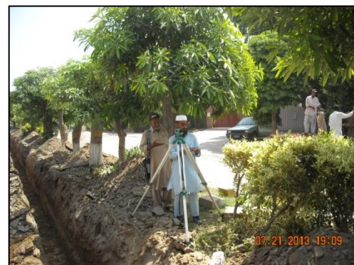
Field verification of levels during construction
